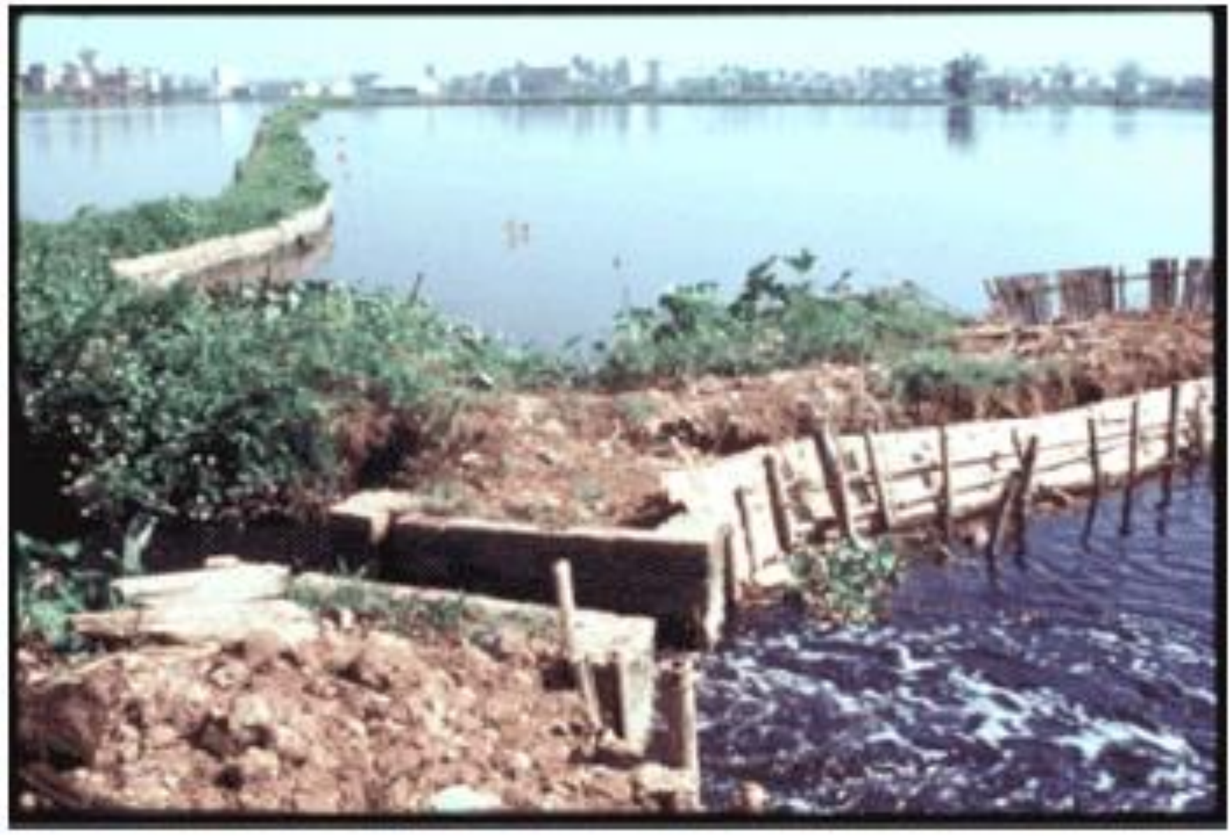
Figure 4: Raw Wastewater and Stormwater Fish Pond in Hanoi City
